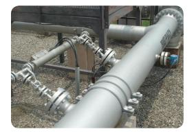
Micro Motion Coriolis and dedicated density meters are ideal for real-time process monitoring, quality control and custody transfer applications
